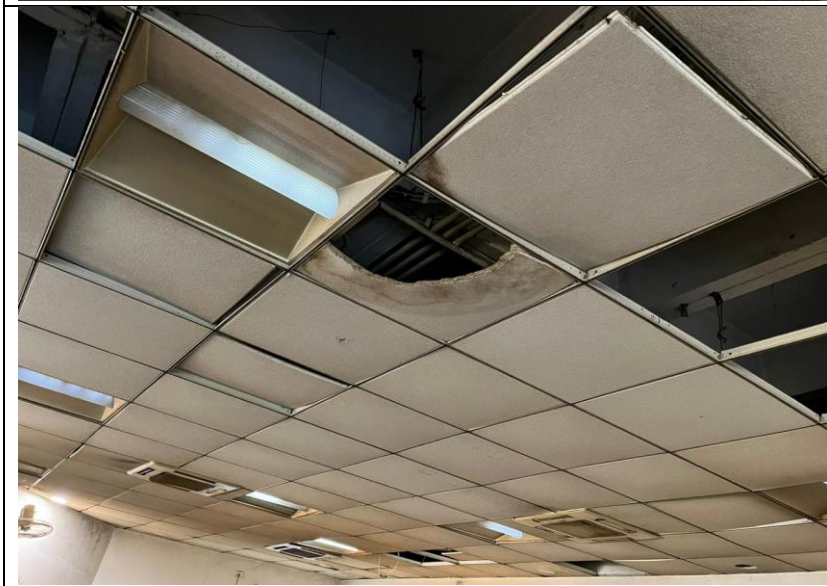
False Roof of Sitting Area
