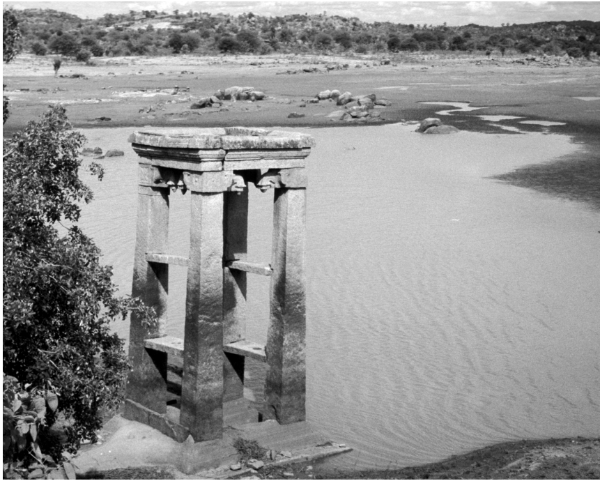
Figure 3. Sixteenth century Timmalapura reservoir with its massive double sluice. Unlike reservoirs to the south and east of the city of Vijayanagara, this reservoir southwest of the city has only had minor silt deposition and is still in use. Photo taken in January.
